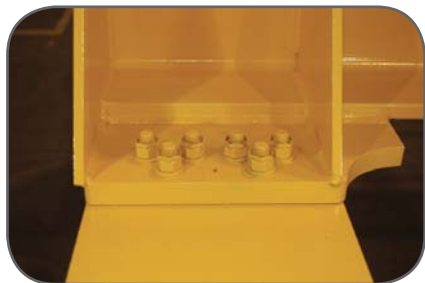
Standard bolted girder connection plates
